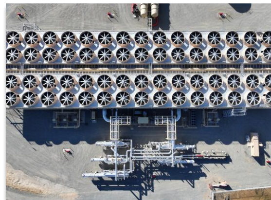
Unit 1 mechanical completion
