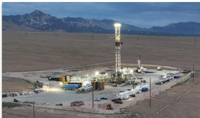
Drilling and completions operations
